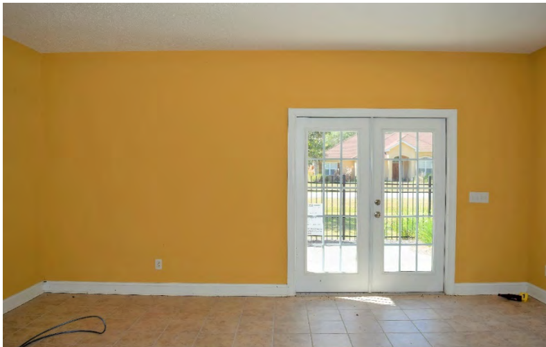
Interior overall photograph of the west wall of the clubhouse.
