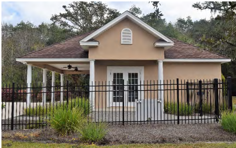
Exterior overall photograph of the east wall of the clubhouse.
