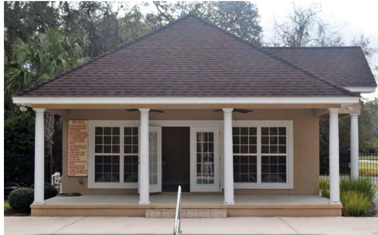
Exterior overall photograph of the north wall of the clubhouse.
